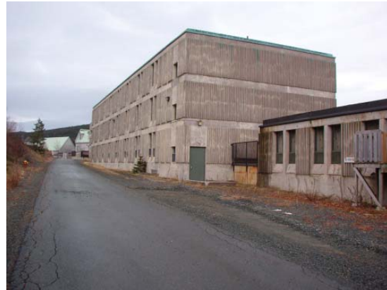
rear façade, north side
