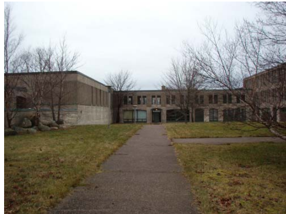
central courtyard east, administration office at center, gym at left, classrooms at right
