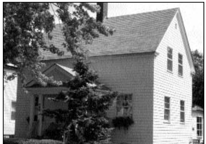
Figure 13: 28 East Valley Road.
