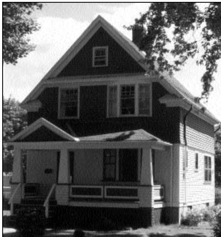
Figure 15: 40 East Valley Road.
