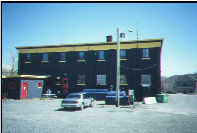
Fire Station, rear facade
