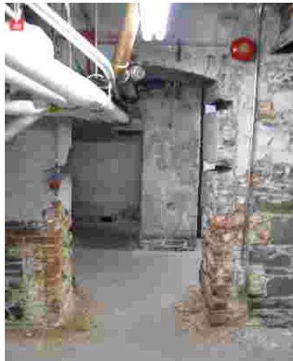
Dungeon showing arched doorways with cells on both side. Note original exposed brick which is decaying, April 2008 © Deborah O'Rielly/ HFNL
